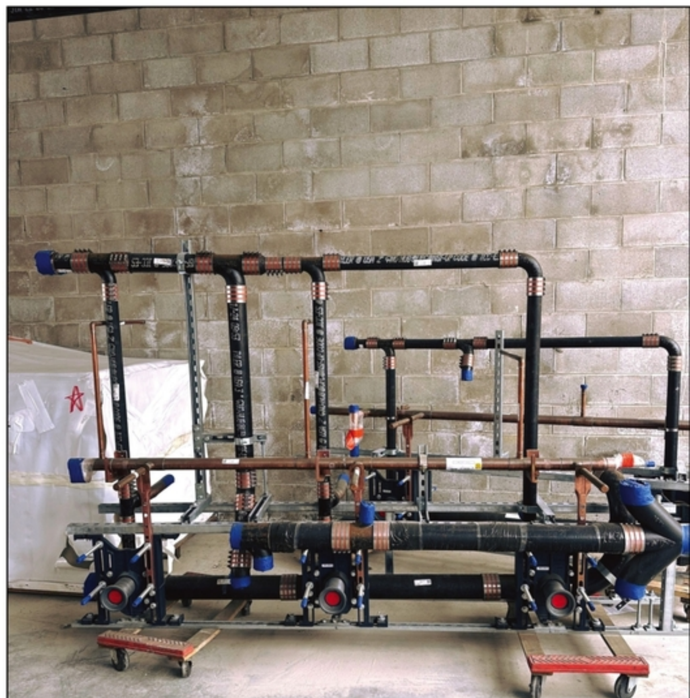
A prefabricated system of plumbing carriers installed by Progressive Mechanical, Inc. illustrates the precision and expertise behind the Schaap Center's high-performance facility. Prefabrication not only reduced install time and waste, but also helped maintain quality control on such an important project. Photo courtesy of Progressive Mechanical, Inc.
